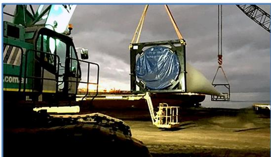
According to Qube, the loads have included lifting and transporting 149 turbine units made up of base towers, nacelle, generator, hub and blades. The heaviest component weighed 110 tonnes while the longest was the top tower at almost 25 metres.
